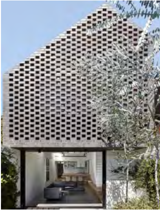
HIT AND MISS BRICK WALL DETAIL EXAMPLES
