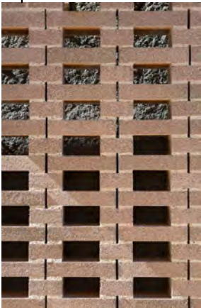
HIT AND MISS BRICK WALL DETAIL
