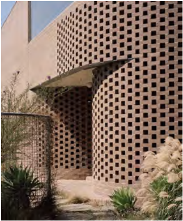
HIT AND MISS BRICK WALL DETAIL EXAMPLES
